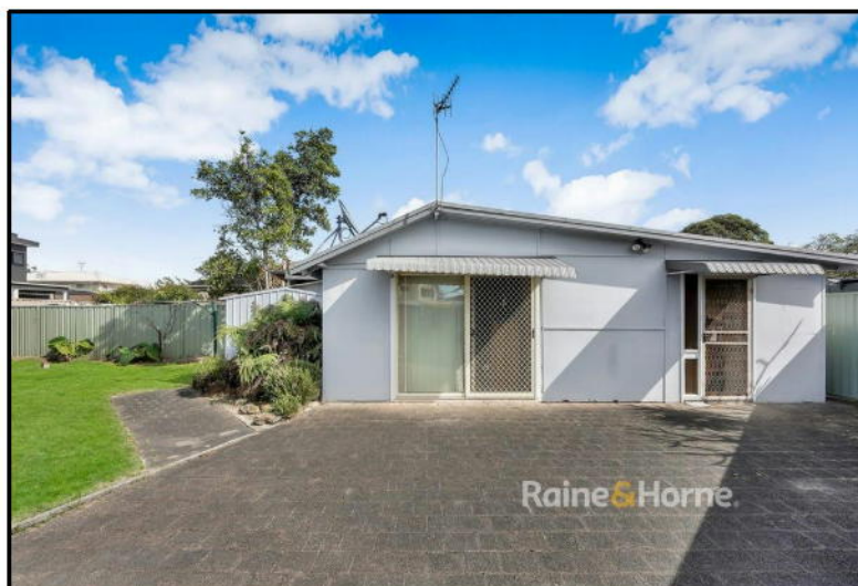
Figure 5: Existing detached studio to the rear of the site addressing the laneway. (Source: realestate.com.au)
