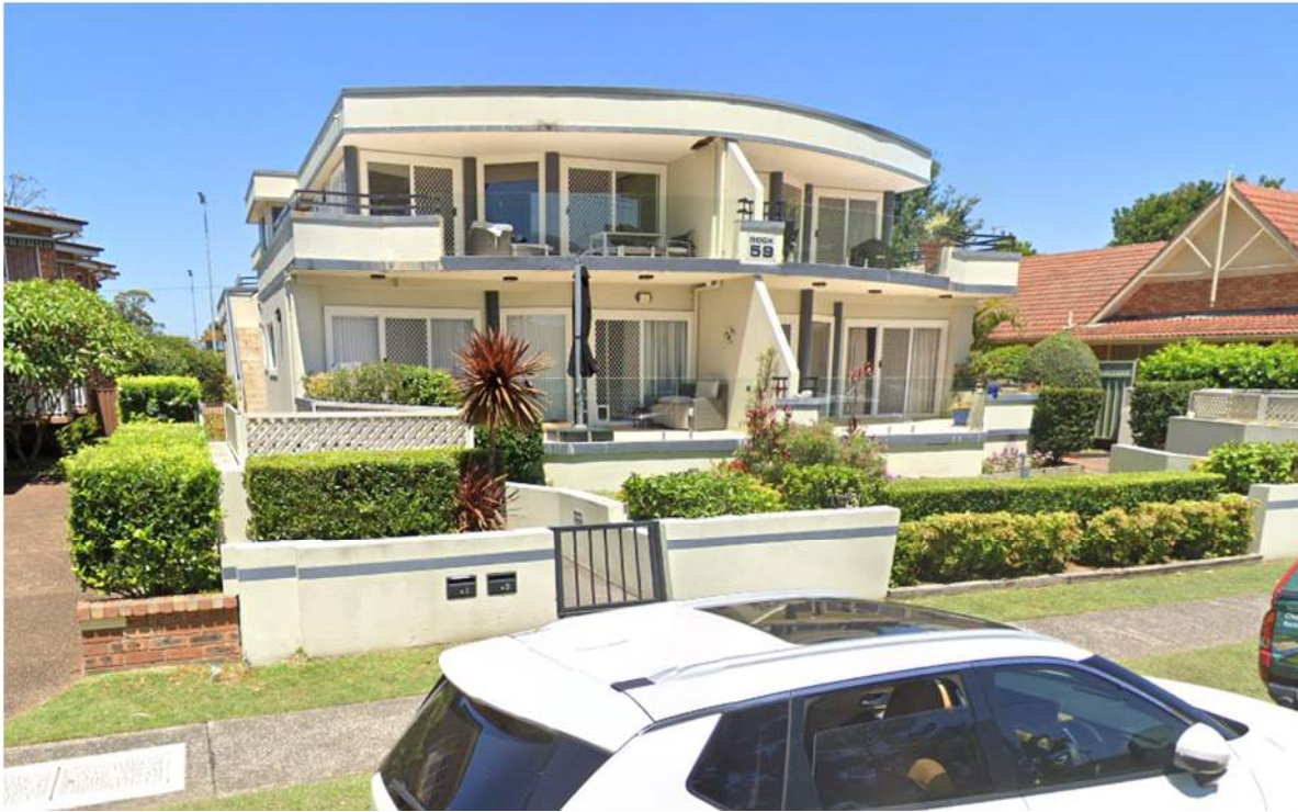
Figure 2 – Existing Manor House viewed from Brick Wharf Rd
