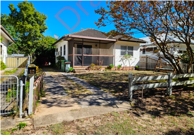
Photo 3: View of existing front façade
