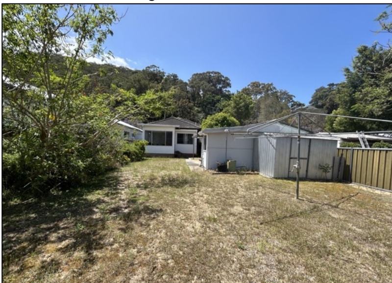
Photo 4: View of existing rear façade
