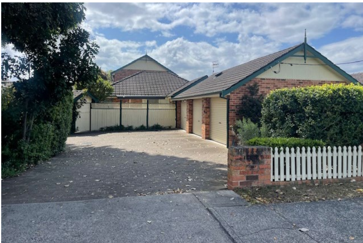
Figure 6. Photo of 185 West Street
