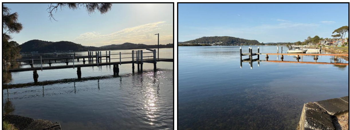
FIGURE 5. Existing and surrounding water facilities to the north (L) and to the south (R)
