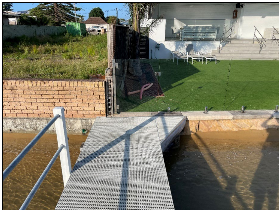
Figure 4 – splayed end to jetty (BIC)
