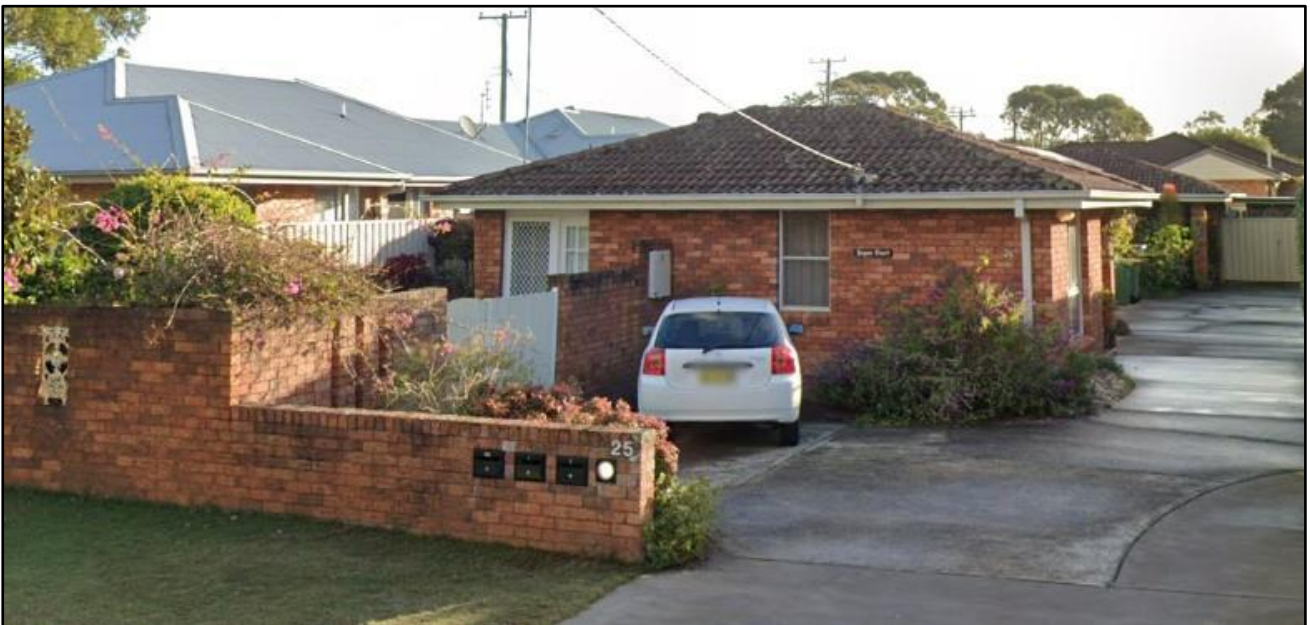
Figure 7. Opposite side of the street
