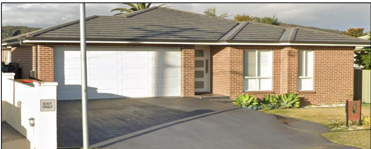
Figure 5. Dwelling House – austere character established
