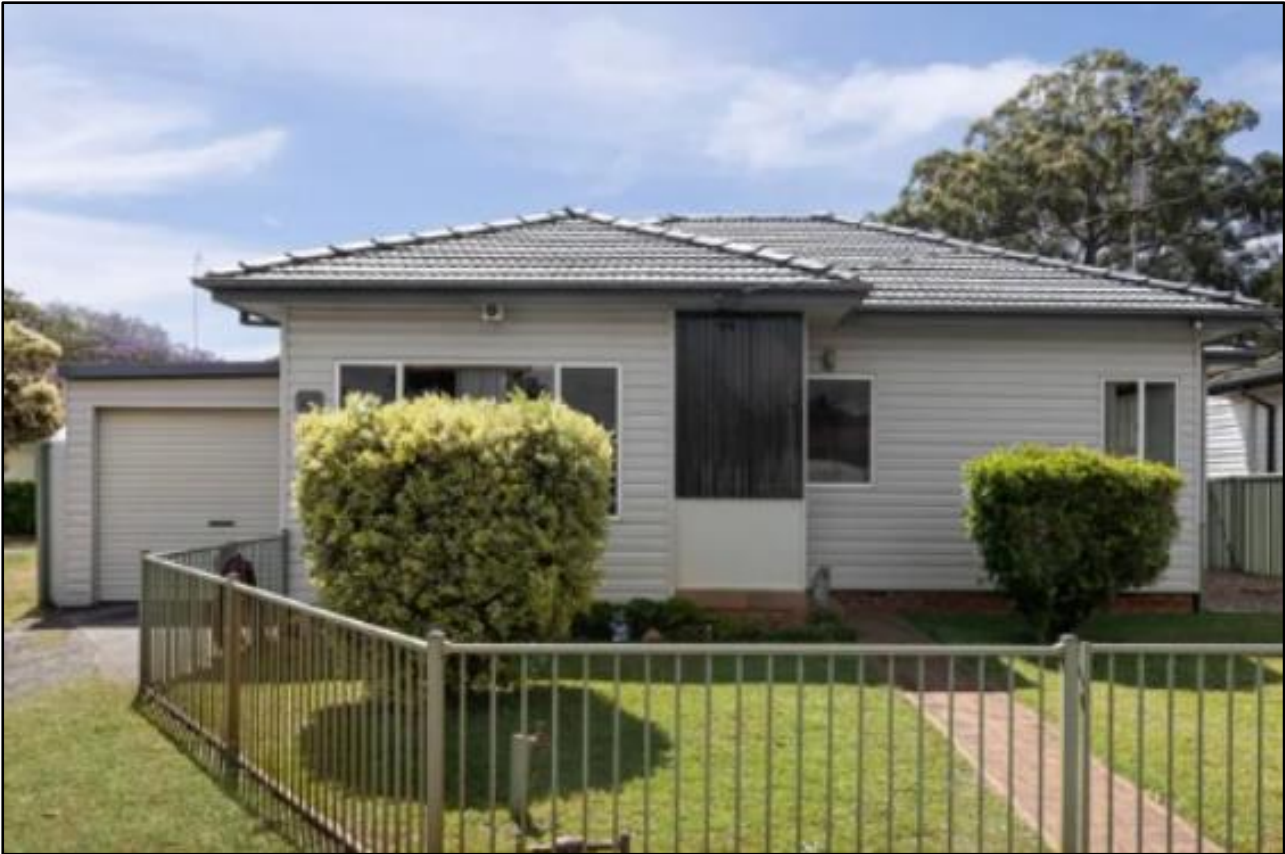
Figure 2. View of the existing dwelling-house viewed from the street
