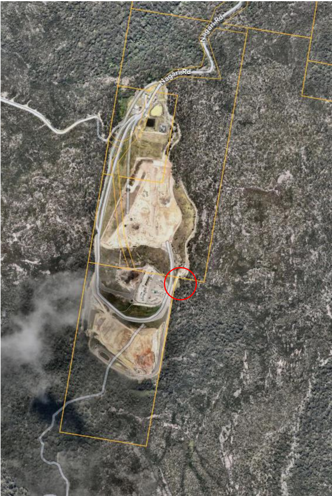
Figure 2 – Location of possible encroachment onto BWNP (source: Nearmap, 29 October 2023)
